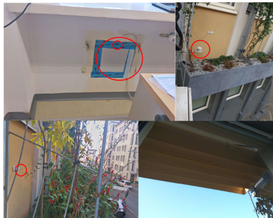
Measuring areas and sensors in/around the room BZ.13 ©Korjenic et al
